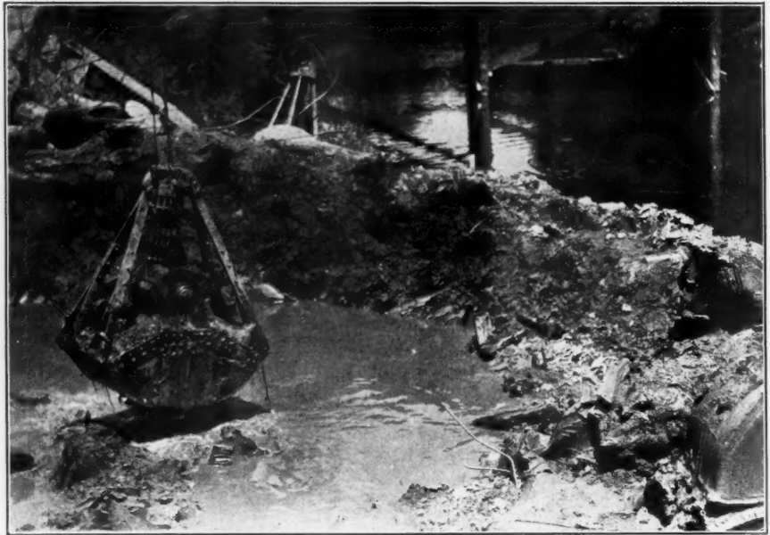
Clamshell Used in Excavating
